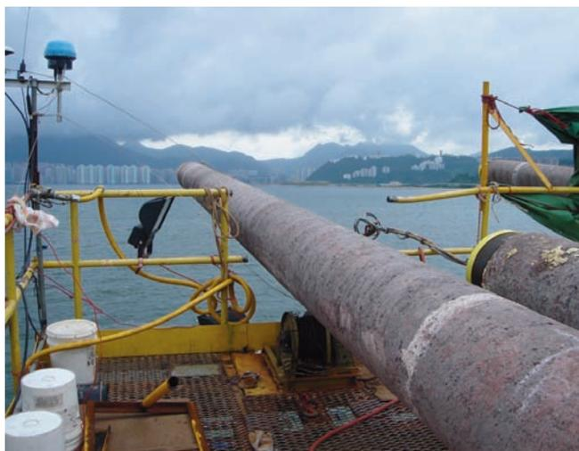
**Figure 4.** This photo from a separate project portrays the typical configuration of the pipe on the laybarge in similar work conditions.
