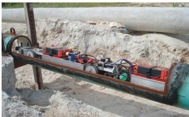
Figure 2. A train of robotic equipment enters a string of pipe to internally coat part of Project A.
